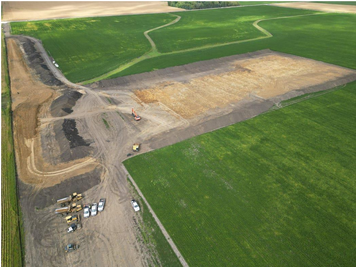
Figure 6: Sept. 7, 2023, berm being built by CRWD in Dobbins Creek.
